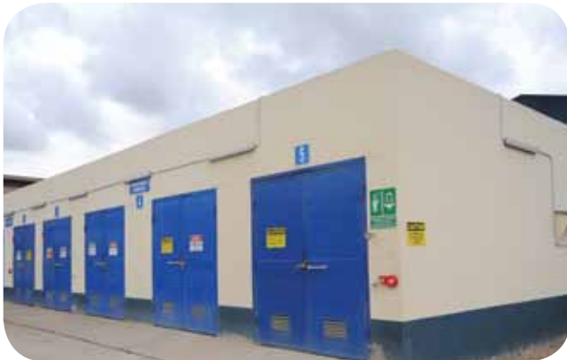
Newly constructed hazardous chemical warehouse will ensure proper handling of chemicals used in our operations.
