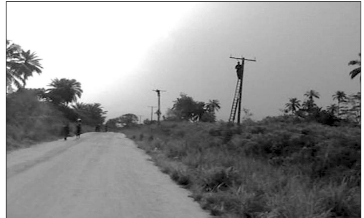
Erection of electricity poles/stringing in Obumeze Community
