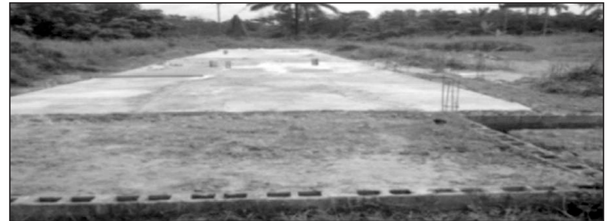
The Foundation of the Rumuekpe Secondary School
