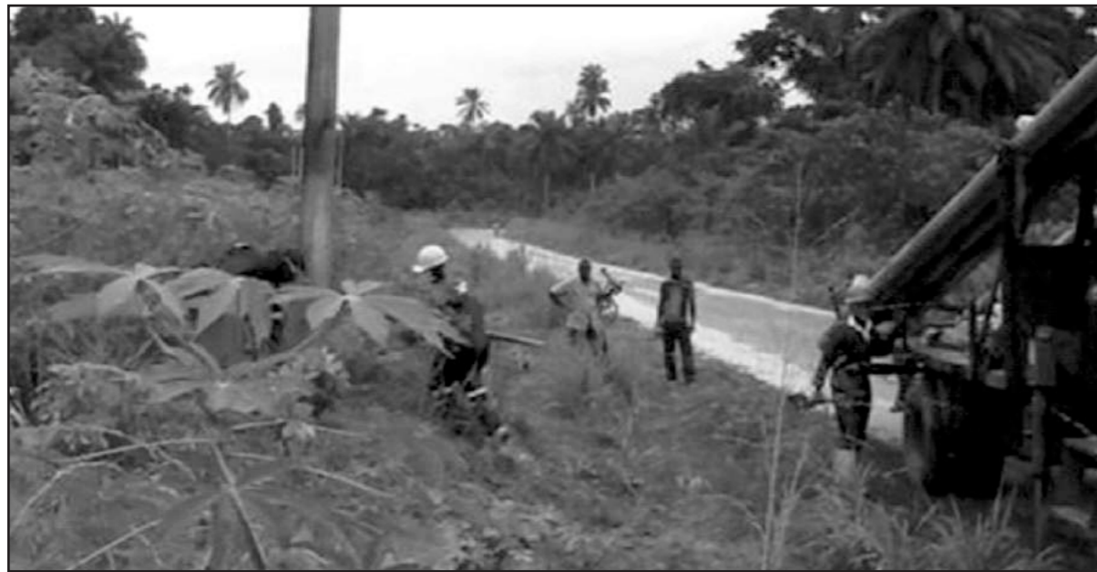
Laying/erection of electricity poles in Ogbele Community
