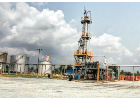
NDPR Mini-Refinery, Ogbele
