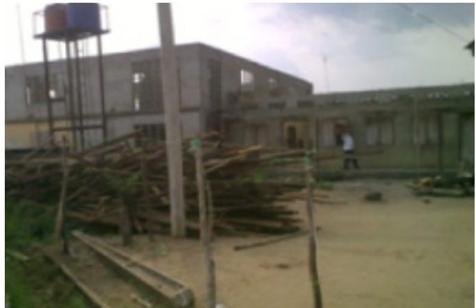
The present Otari Community Town Hall de-roofed
