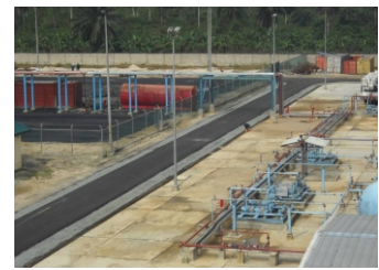
Inside the Ogebe Flowstation
