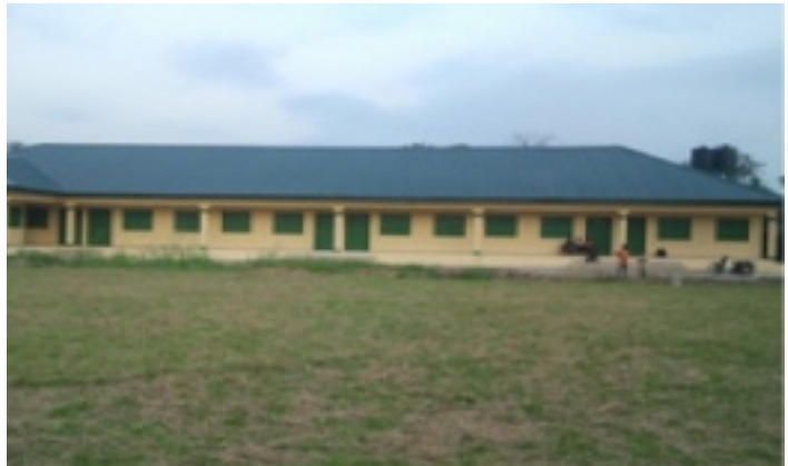
North View of completed School at Obumeze
