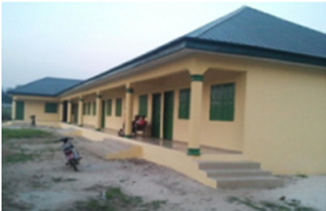
Completed Obumeze Primary School
