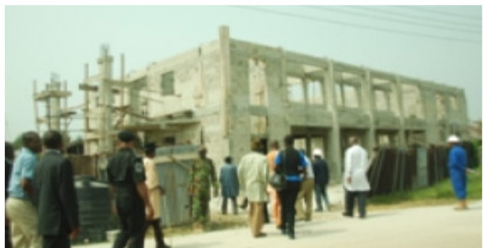
Renovation work in progress
